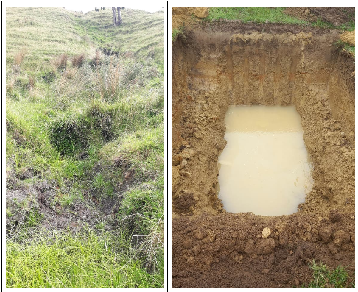
Photograph 4.8a&b: (a) Groundwater seeps from gullies resulting in shallow landslides and (b) in test pits along the soil / rock interface
